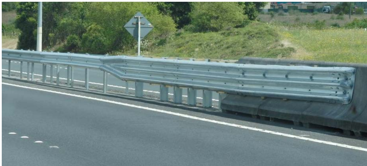
Nu-Guard-31™ Transition To A Thrie-Beam Bridge Connection
