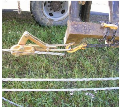
Vehicle Cable Pull
