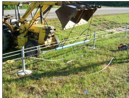
Hydraulic Cable Pull
