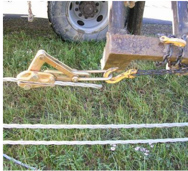
Vehicle Cable Pull
