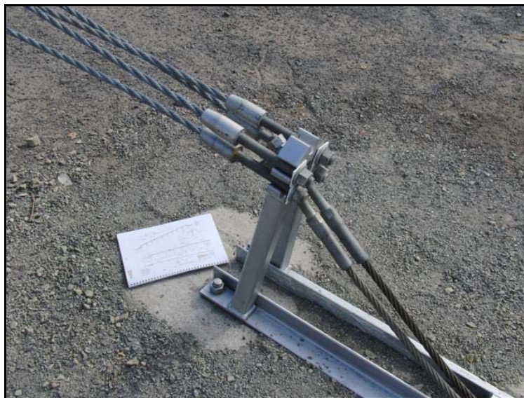
NU-TEN® TERMINAL END connected to a 4 cable barrier*
